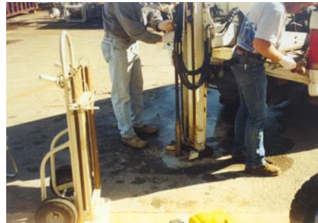
Geoprobe rig at the facility
