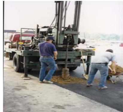
Installation of Well
